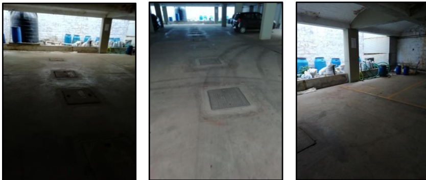
Figure 1. Examples of small scale sewage treatment plants.
