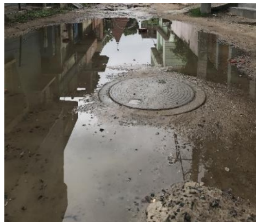
Figure 1: Sewer network manhole in water logged area (Harsh/NU/2019).
