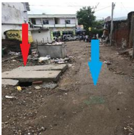
Figure 2: Old and new sewer in ward 11 (Harsh/NU/2019).
