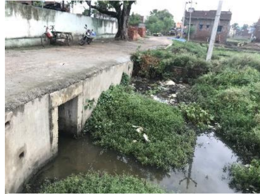
Figure 11: Treated effluent from STP and storm water drain opening to a Pyne (Harsh/NU/2019).
