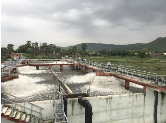
Figure 10: Sewage Treatment Plant in Rajgir (Harsh/NU/2019).
