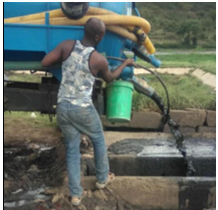
Figure 7 Mechanical emptying is generally safer than manual emptying but significant hazards remain without operating procedures that emphasise health and safety. Picture credit: SNV
