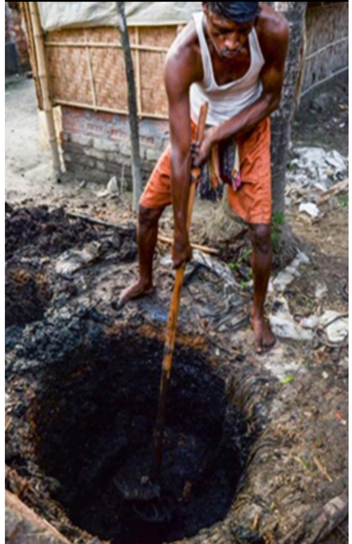
Figure 1 Manual emptier working without protection. Picture credit: SNV
