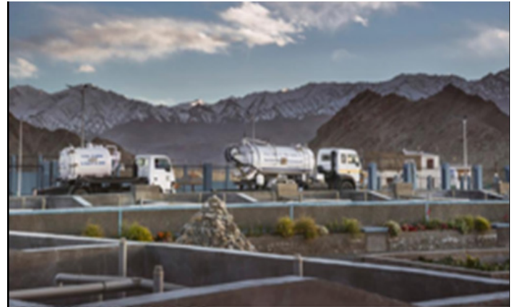
Figure 1 Blue Water Company vacuum tankers arrive to discharge sludge at the faecal sludge treatment works the company funded, built and operated in Leh, North India. Picture credit: Spalgon, R.
