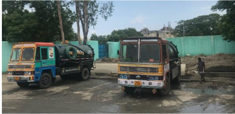
Figure 6: Septage lorries decanting at Nesapakkam STP (Kripa/Eawag/2019).
