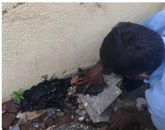
Figure 9 : A sanitation worker preparing to clean an LIO in North Region, GCC (Kripa/Eawag/2019).
