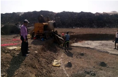
Under Construction FSTP site in Sinnar
