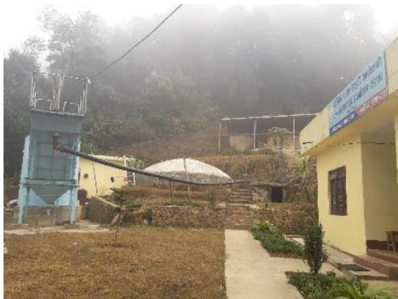
Figure 8: Office building and Various Units of Waling Small Town Water Supply Scheme
