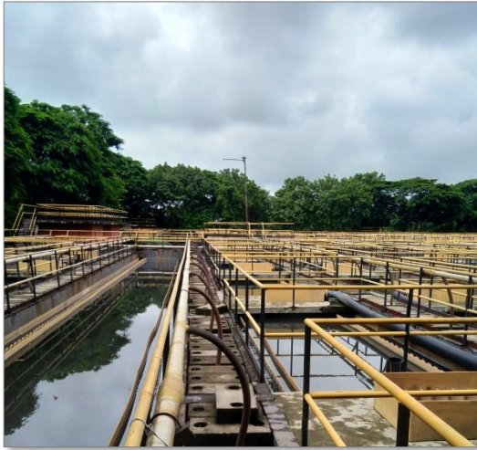
Figure 3: STP of 78 MLD capacity with UASB technology
