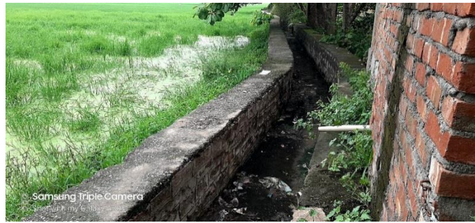
Figure 4: Conveyance of wastewater and supernatant through open drain (Manish/CSE,2020)
