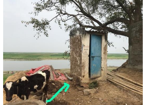
Figure 3: Household in ward 25 (vicinity to Ganga river) had toilet directly connected to drain (Source: Harsh/CSE, 2020)
