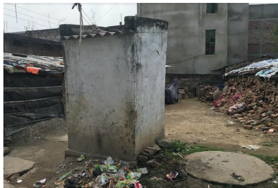
Figure 4: Fully Lined Tank and Lined Pit impermeable wall and open bottom (Source: Harsh/CSE, 2020)
