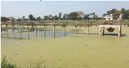
Figure 2: Existing STP of 11 MLD Capacity (Source: Shrutaswinee/CSE 2020)
