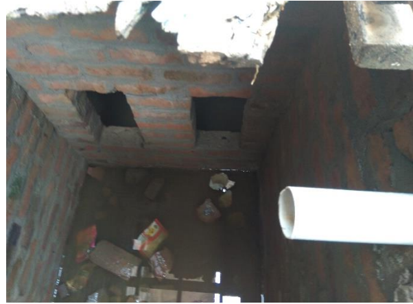
Figure 2: Under construction 2 chambered septic tank
