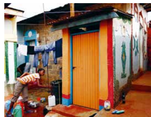
Upsized toilet facility, Kenya
