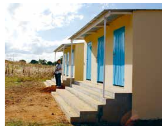
School sanitation facility, Zambia
