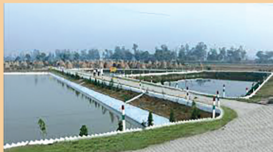
Waste stabilization pond at Chandsamand village
