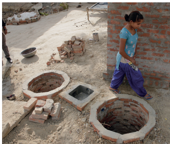
Twin-pit toilet constructed in Gonda, Uttar Pradesh
