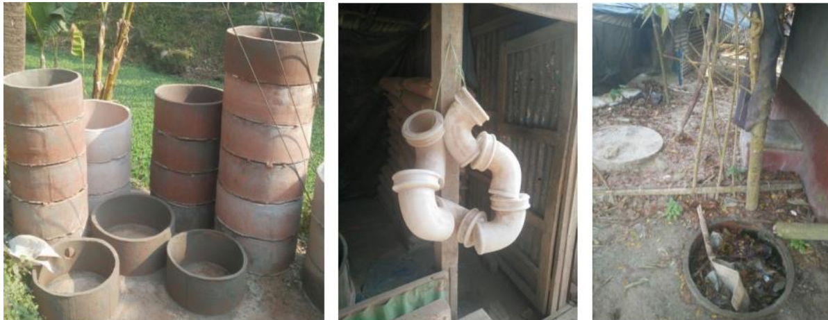
Figure 5: Rings used for pit containment and siphons made in Bhola and backside of toilet with a double pit (Source: UPM 2020).
