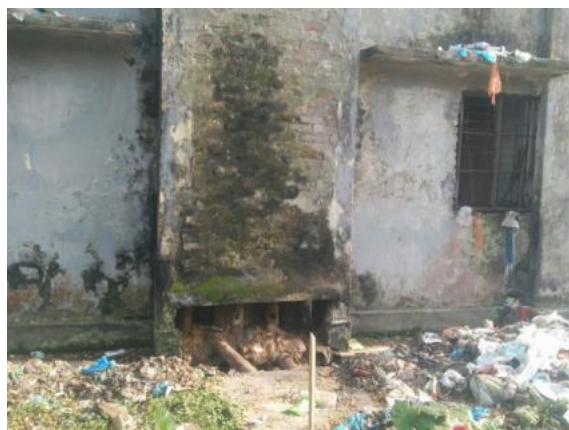
Figure 10: Discharge into open drain at the backside of Bhola public hospital (Source: UPM 2020).
