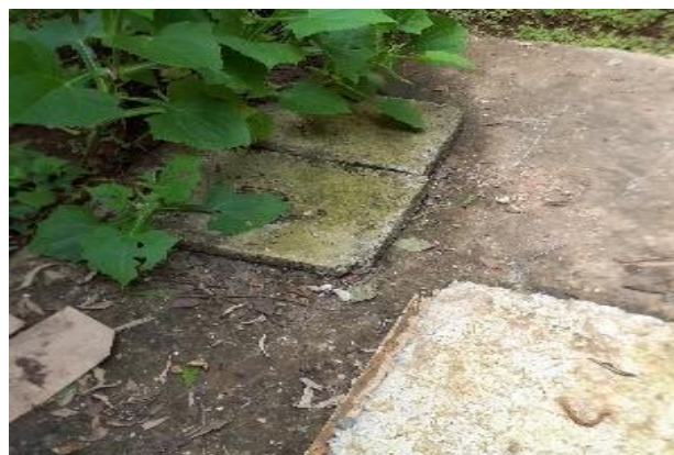
Figure 2: Containment system (HHs Survey, 2019).
