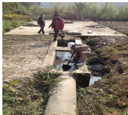
Figure 3: Decentralized Wastewater Treatment System.
