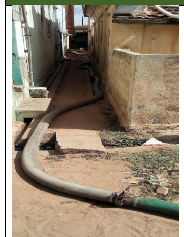
Figure 3.3: Narrow Lane De-sludging at E. Pudhur
