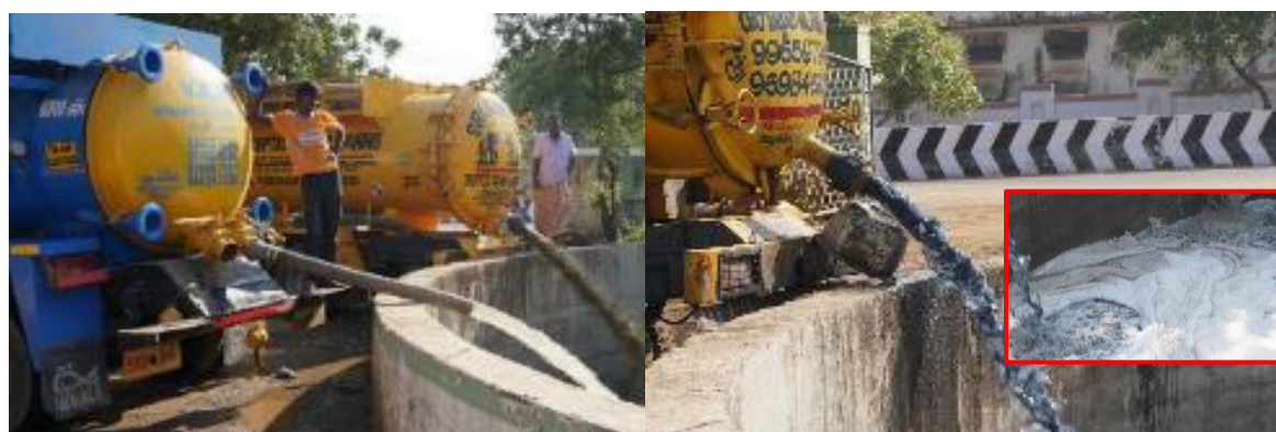
Figure 4.15: FS Disposal with No PPE and Non-Domestic Source of Sewage Discharging
