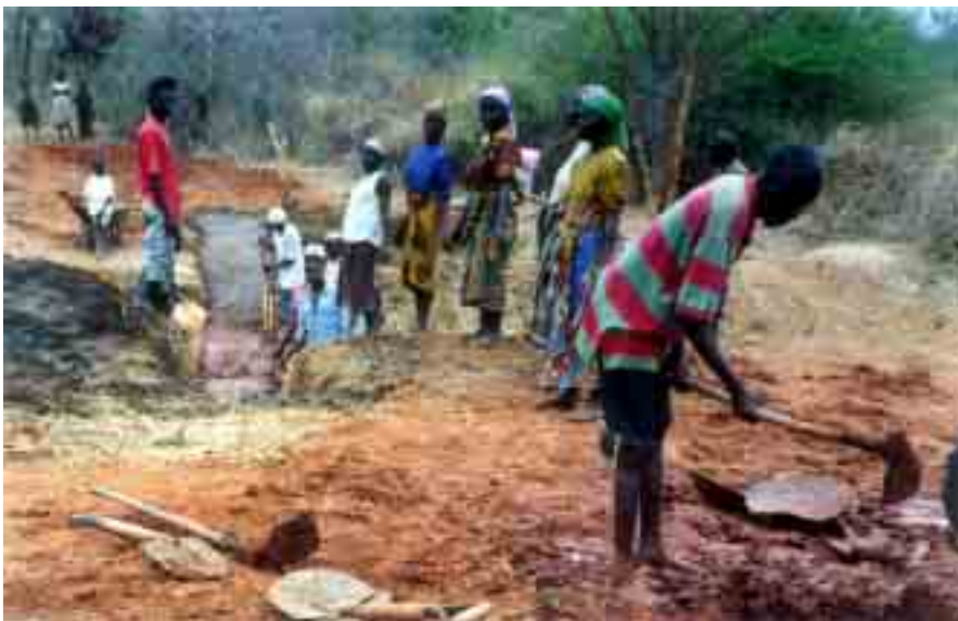
Plate 3: A community building their subsurface dam of soil.
