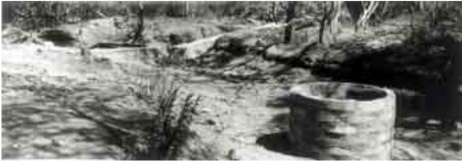
Plate 4: A hand-dug well with a subsurface dam downstream.
