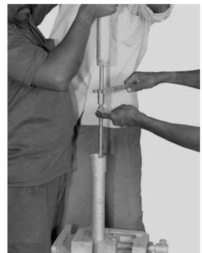
Pumprod opening while holding riser pipe
