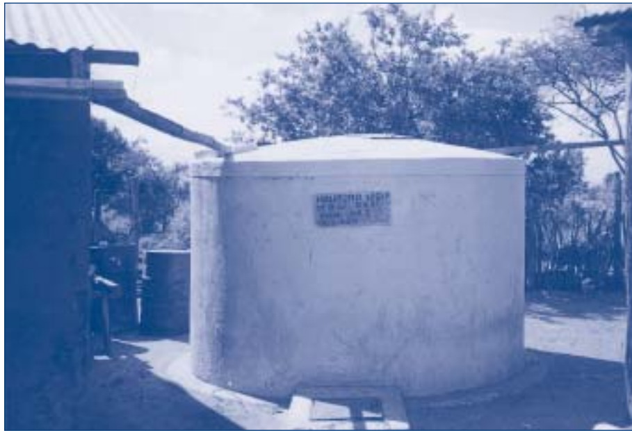
Fig. 7.1. Simple roof catchment and storage
