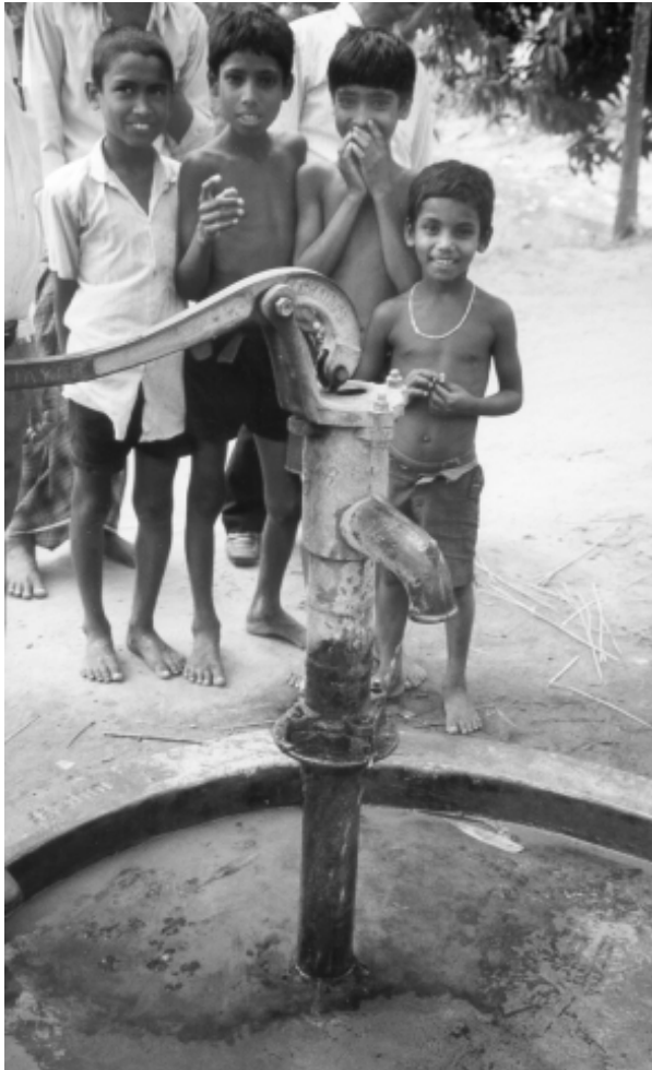
Figure 19 Suction Pump
