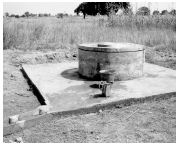
Figure 10 Hand-dug well
