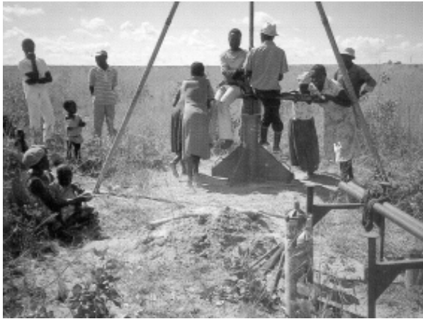
Figure 11 Hand drilling
