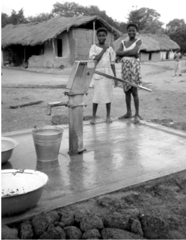
Figure 24 Deep Well Pump
