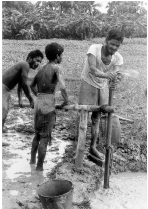
Figure 14 Hand drilling with sludger method
