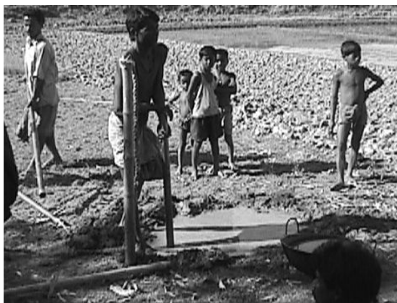
Figure 4: Mistry Starting a Hole with 1.5m Pipe
