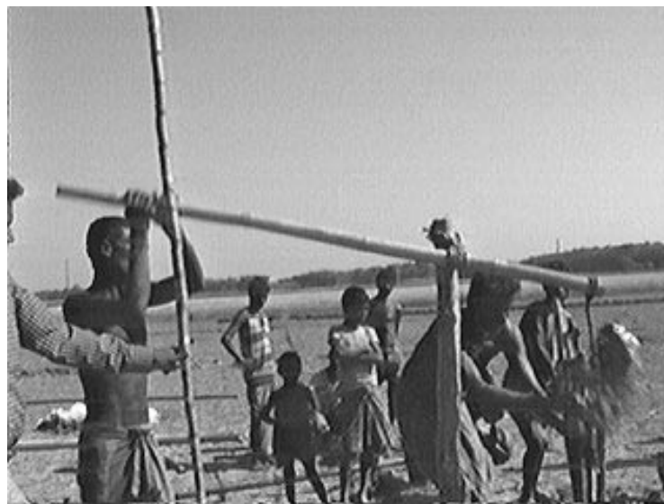
Figure 1: Mistries Operating Sludging Equipment
