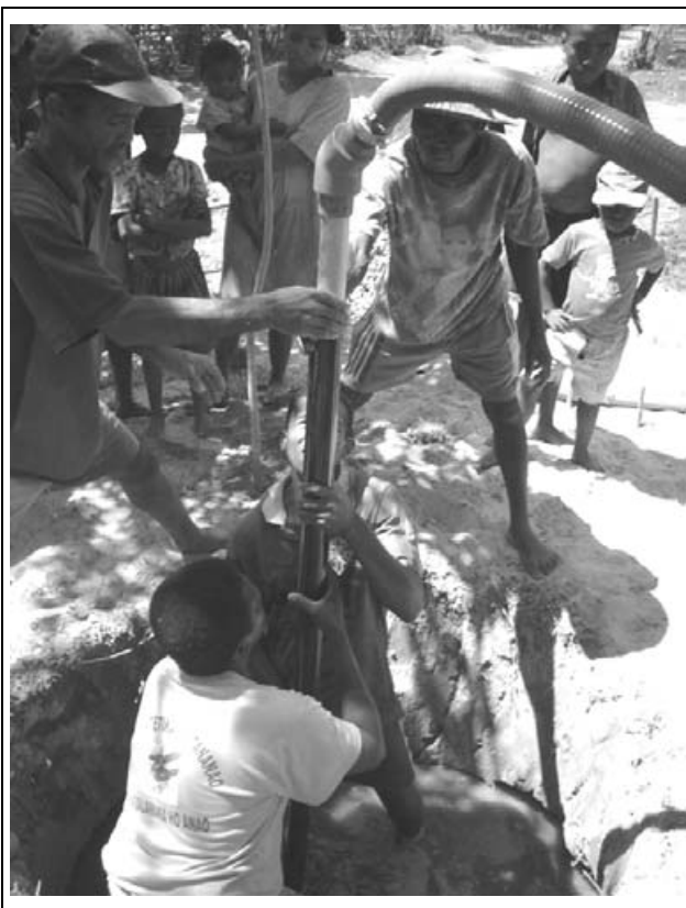
Photograph 1. It only takes about 2 minutes to jet a well screen 4-5 meters into the aquifer.
