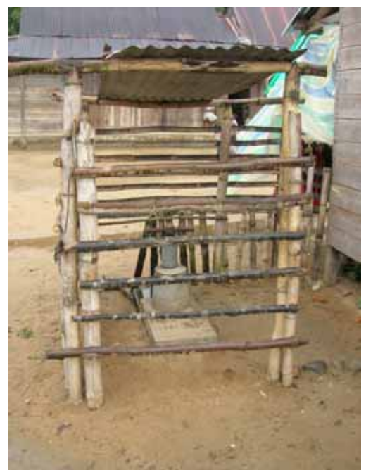
Mahalevona MV 18, too close to house
