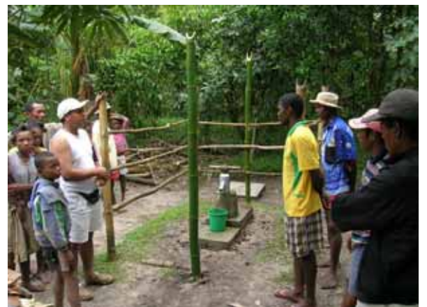
Antoraka AT 15, roof is detachable, see also washing slab (background)
