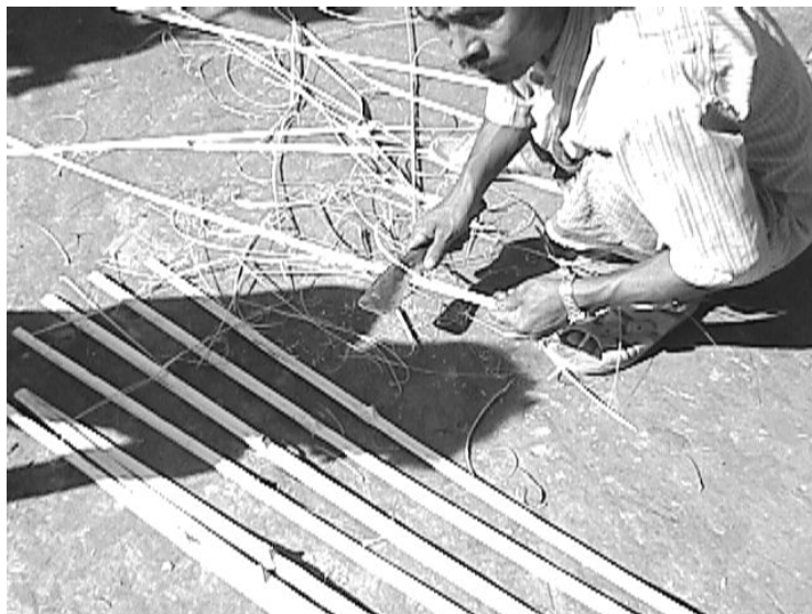
Figure 11: Cutting of Bamboo Slats
