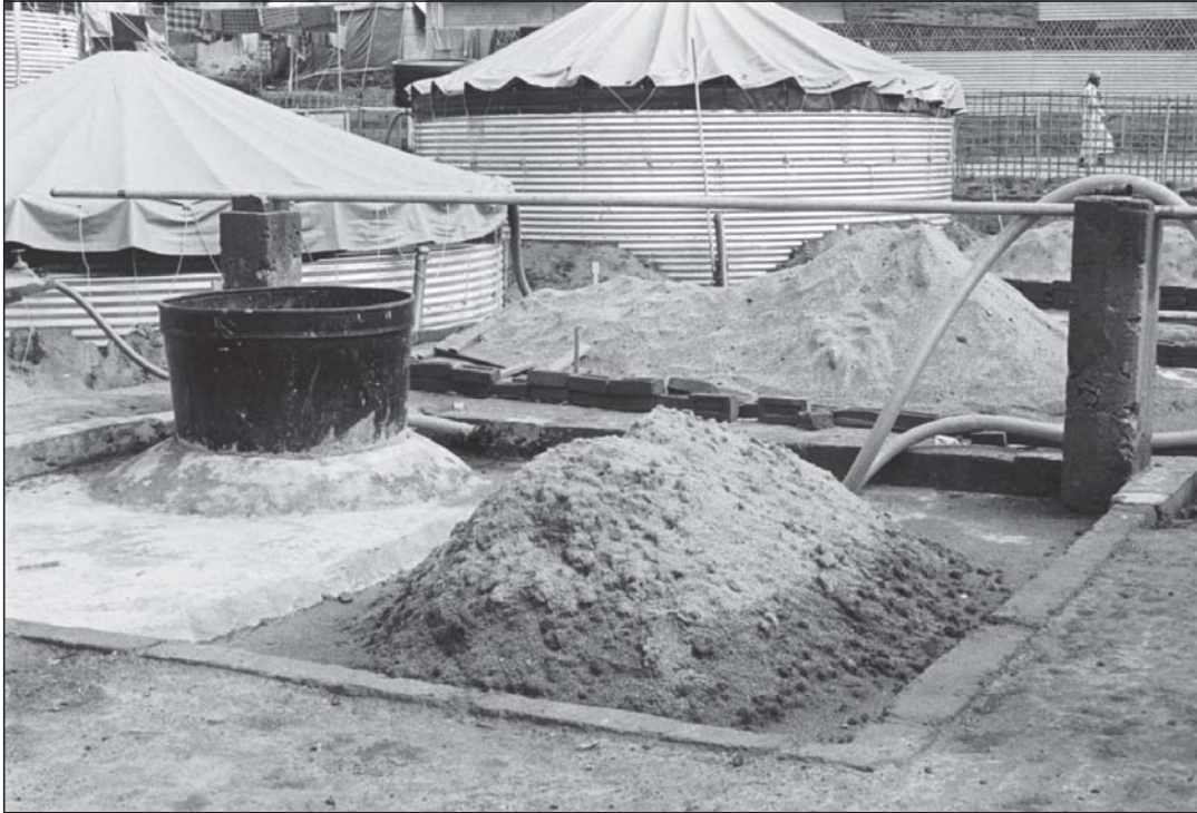
Above: Sand cleaning for slow sand filter, Dumdumia Refugee Camp, Bangladesh Below: Mobile water treatment units, Rwanda
