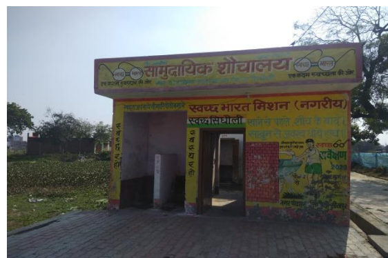
Figure 4: Community toilet constructed under SBM (U) (Source: Naveen/CSE/2020).
