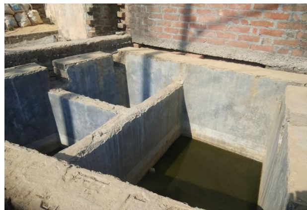
Figure 3: Septic tank under construction (Source: Naveen/CSE/2020).
