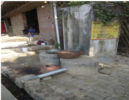
Figure 2: Two chambered circular septic tank (Source: Naveen/CSE/2020).
