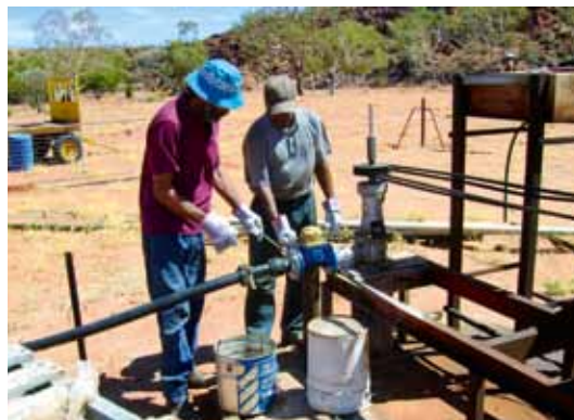
As part of the improvement plan, a water meter is being installed by community members in Australia. Prior to the WSP, the community had no effective means to measure the amount of water they were using.
