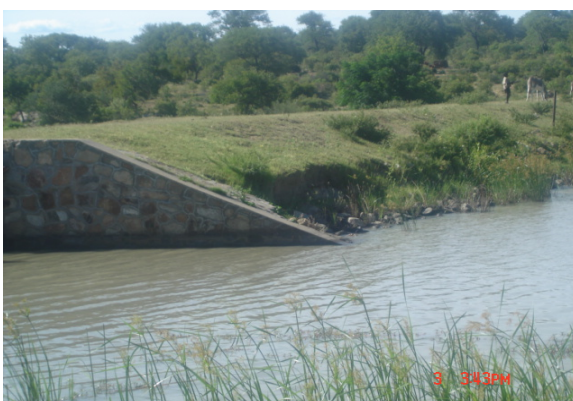
Picture 5. Scarping at Hlashtwayo dam
