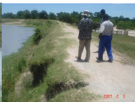
Picture 6. Scarping at Embondweni dam
