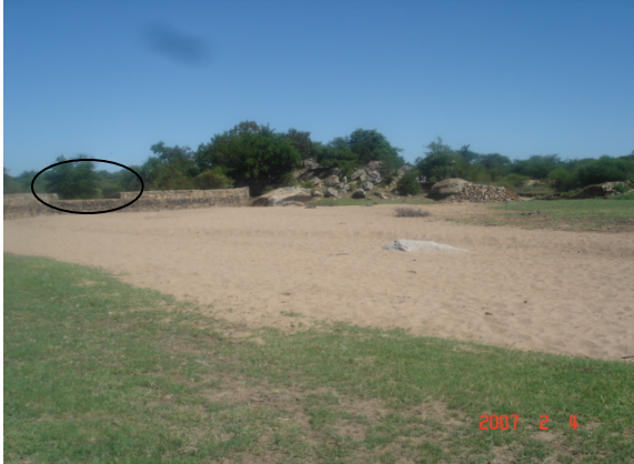
Picture 7. Siltation at Chobhukwa dam. The spillway is encircled.
