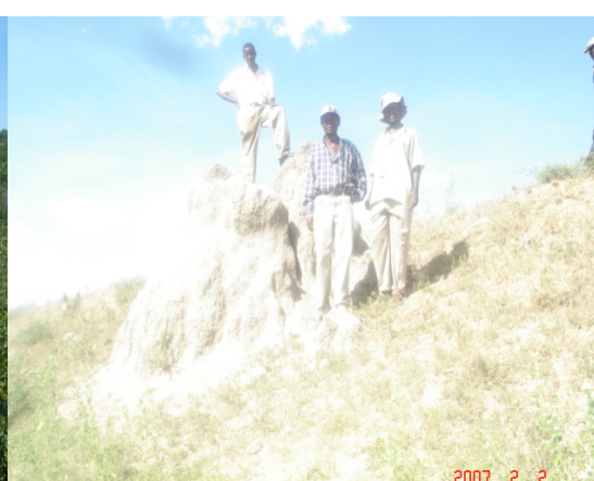
Picture 4. Huge termite mound at Sidzibe dam wall
