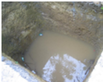
Figure 12. Pit latrines with unlined and brick-lined containment and open bottom, commonly found in Cap-Haïtien
