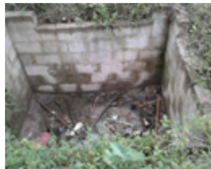
Figure 12. Pit latrines with unlined and brick-lined containment and open bottom, commonly found in Cap-Haïtien
