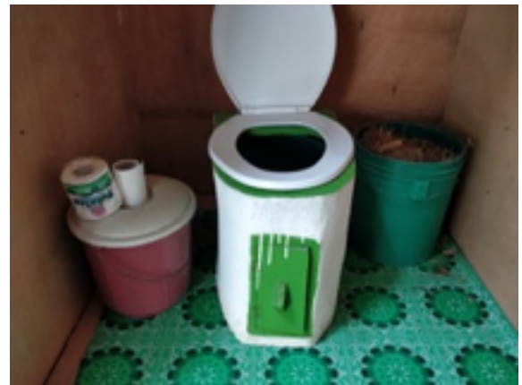
Figure 14. SOIL CBS toilet and cover material (sugarcane bagasse) on the right. Photo credit: SOIL
