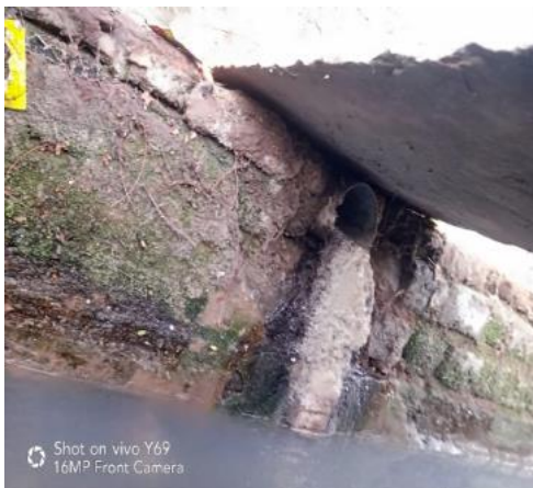
Figure 5: A fully lined tank connected to open drain (Jyoti Parsad/CSE/2020).
