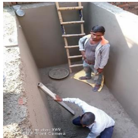
Figure 6: A septic tank under construction (Jyoti Parsad/CSE/2020).
