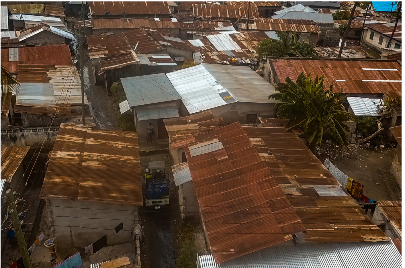
Figure 15 Unplanned area in Dar es Salaam, inaccessible by vacuum truck, partially accessible by motorised tricycle
