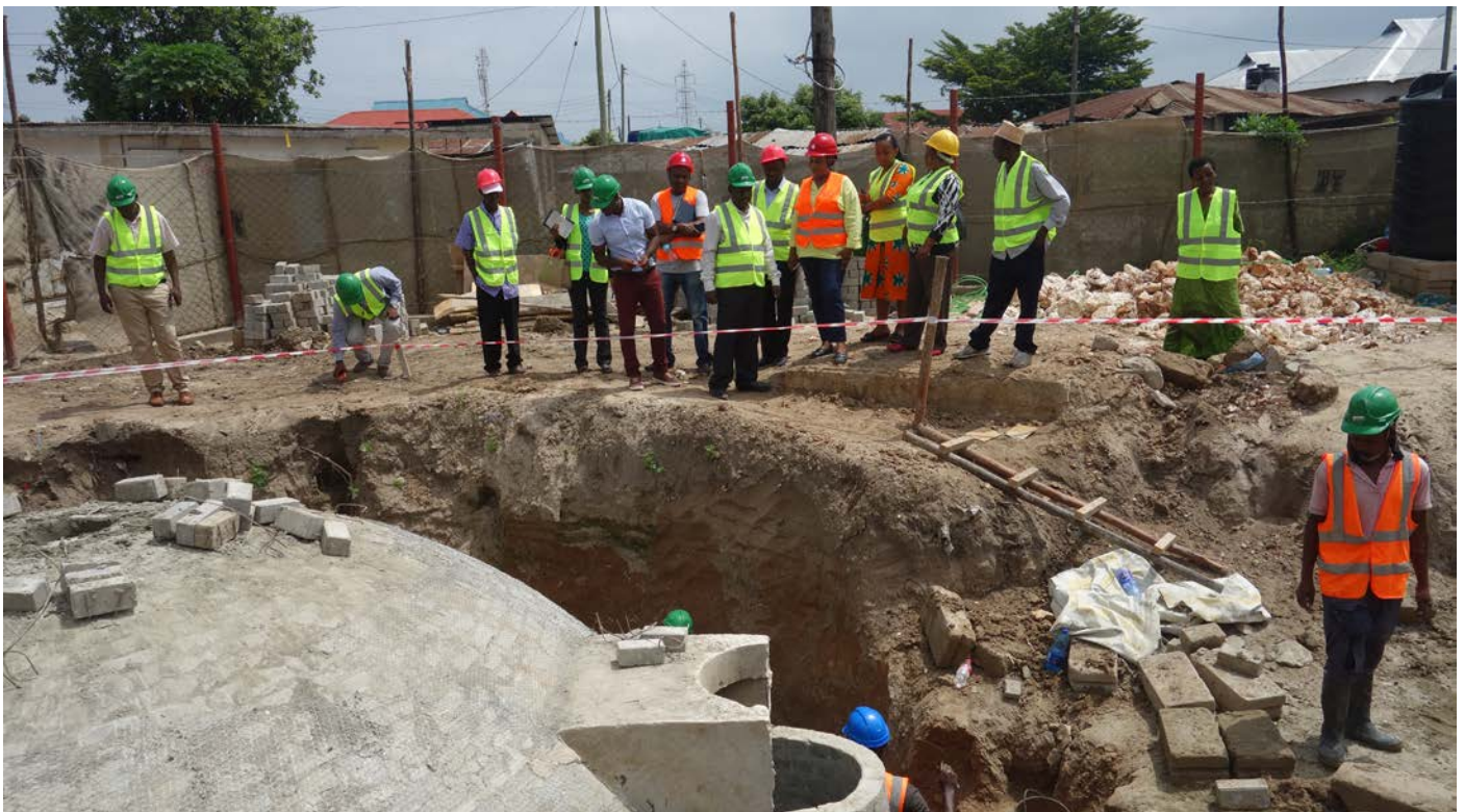
Figure 52 Site visit of key stakeholders during construction of the biogas settler
