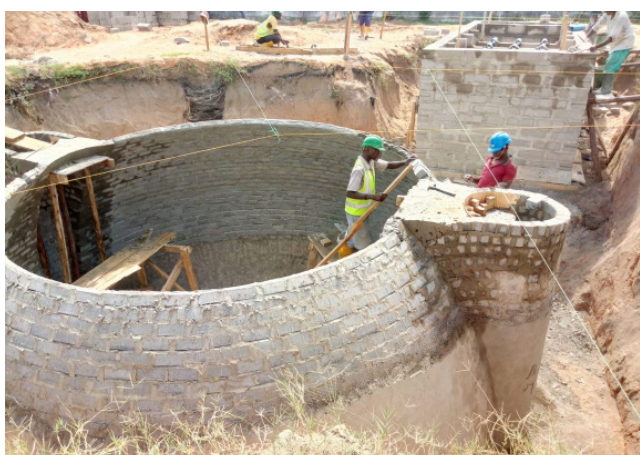
Figure 49 Construction of Biogas Settler
