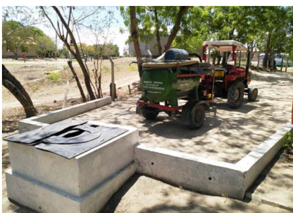
Figure 45 Discharging FS at the Tungji-Kigamboni FSTP with the SludgeGo
