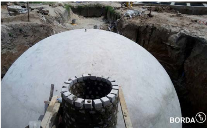
Figure 56 Construction of the Biogas Settler at Mburahati - Ubungo
