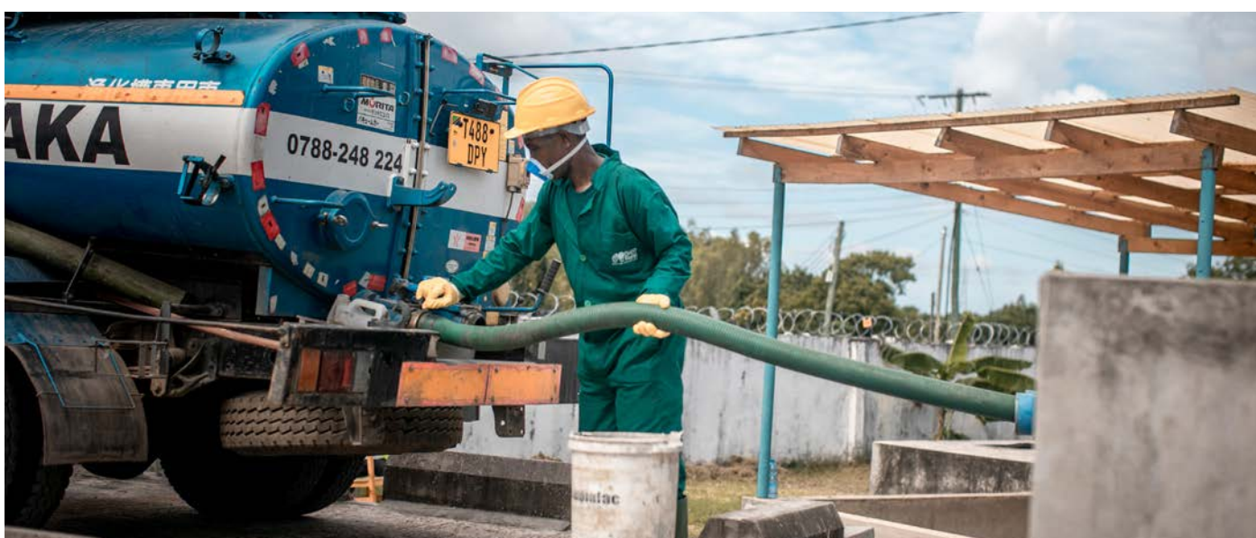
Figure 3 Discharging FS at Miburani-Temeke FSTP, Dar es Salaam
