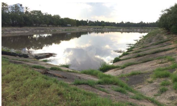
Figure 6 WSP for wastewater treatment in Dar es Salaam
