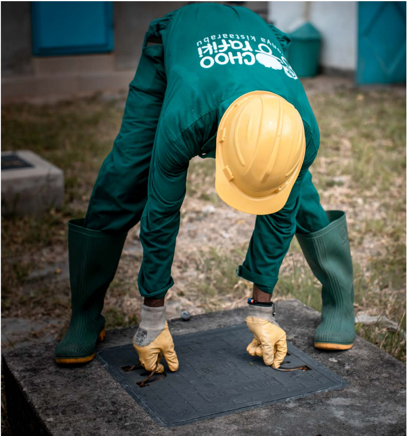
Figure 61 Inspecting manholes at Miburani-Temeke FSTP
