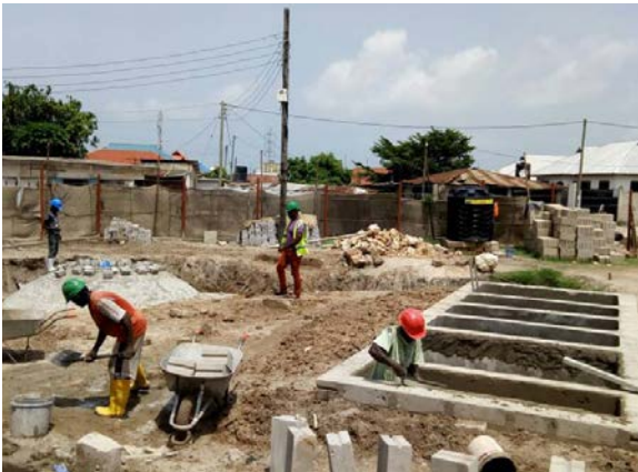
Figure 51 Construction of ABR, AF and Biogas Settler at Mburahati-Ubungo FSTP
