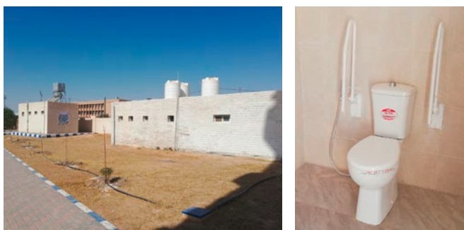
Barrier-free toilet at rehabilitated sanitary facility at Salah Eddin Mosque
