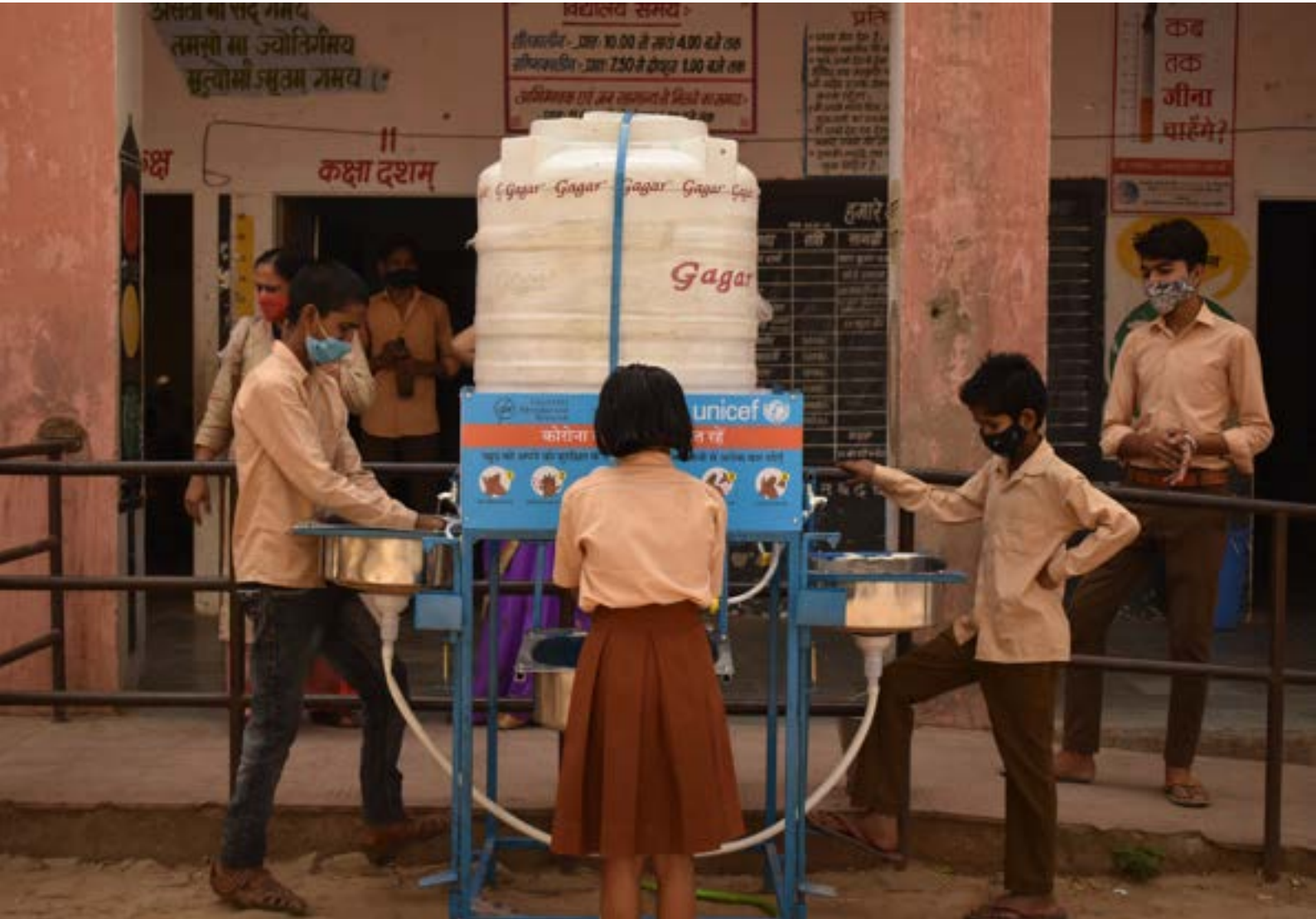
Figure 2: Final design of the handwash station installed
