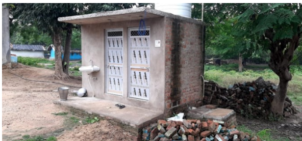
Figure 3: Toilet Connected to Fully Lined Tank (CSE/Manish Mishra, 2021).
