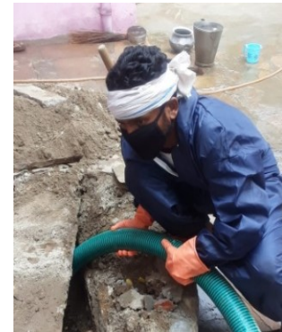
Figure 5: Emptying FS from Sarai Taikore septic Tank (CSE/Manish Mishra) 2021).
