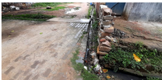
Figure 6: Transportation of Supernatant through open drain (Nullah) (CSE/Manish Mishra, 2021).
