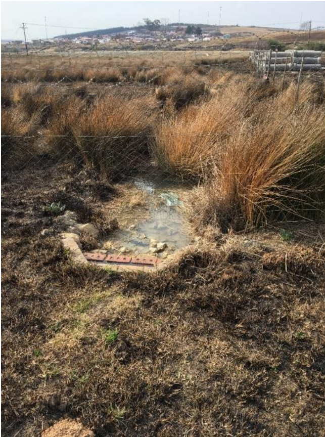
Figure 12: Treated effluent discharge from Prentjiesberg WWTW
