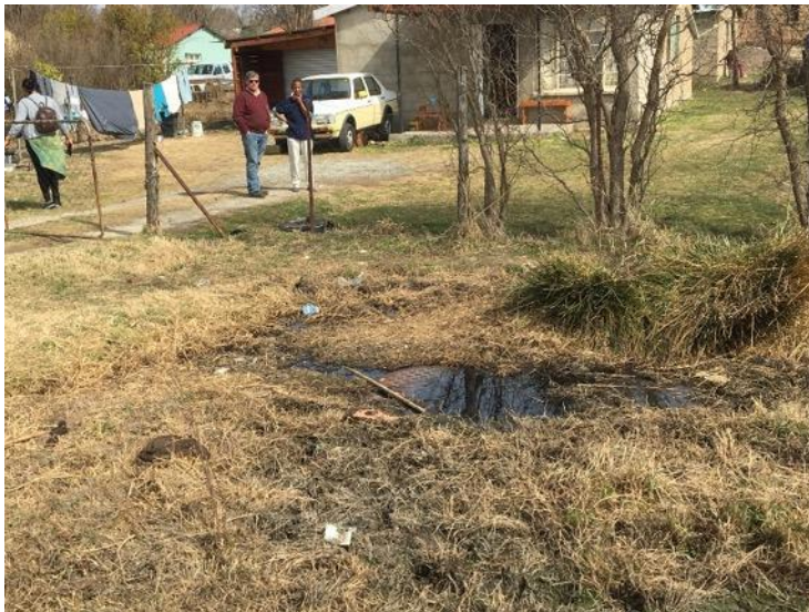
Figure 9: Evidence of poorly constructed and leaking containment tanks
