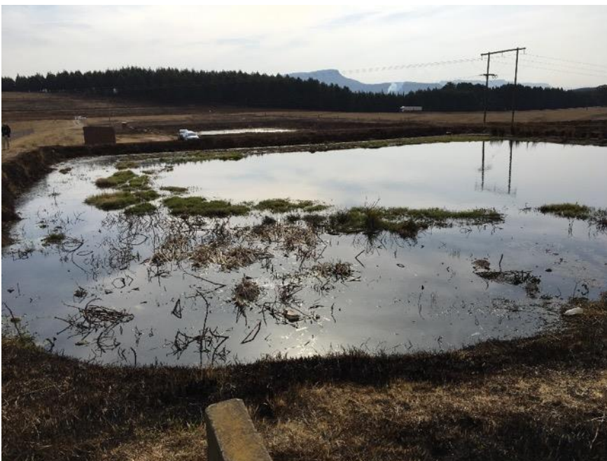
Figure 13: Ugie Ponds showing accumulated sludge
