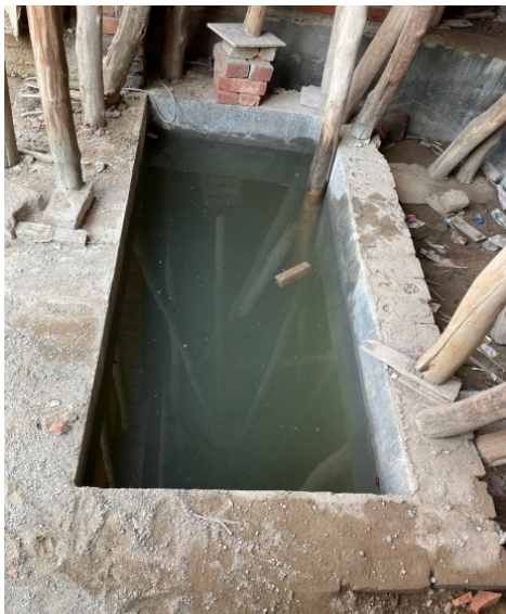
Figure 5: Under construction FLT (Source: Harsh/CSE/2021).
