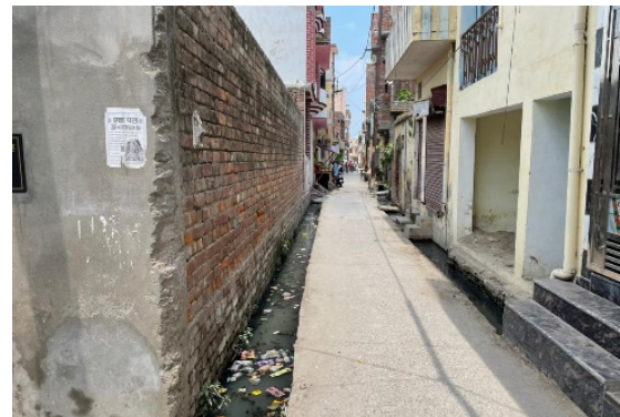
Figure 3: Blockage in open drains (Source: Harsh/CSE/2021).
