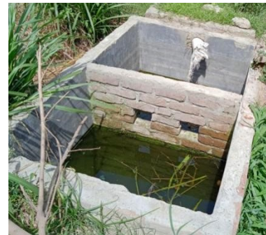
Figure 7: A Septic tank under construction (Aamir/CSE/2021).
