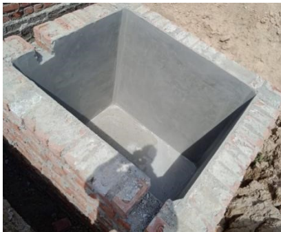
Figure 5: A Fully lined tank under construction. (Aamir/CSE/2021).
