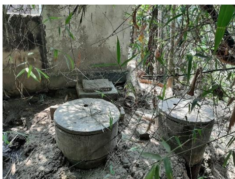
Twin pit latrine
