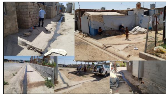
Figure 8: Grey water collection system of channels within Domiz 1 (Source: Author, 2018)
