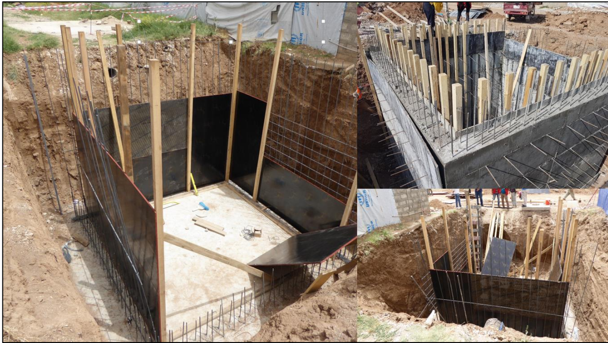
Figure 16: Concrete holding tank, considered fully sealed. (Source: UNHCR Duhok, 2019)
