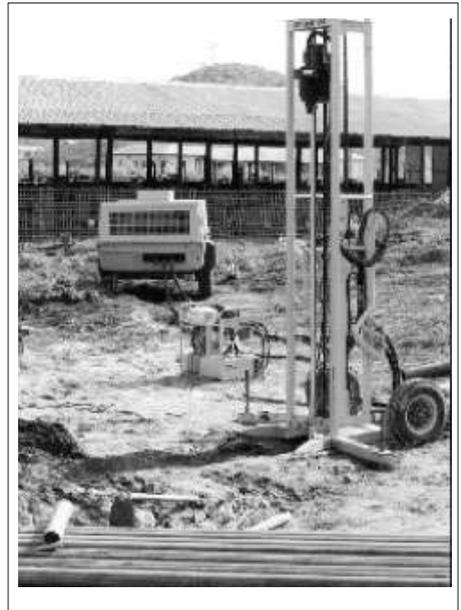
**Figure 7: Rig, hydraulic pump, compressor.**
