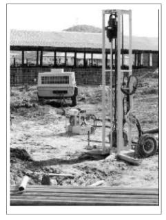
Figure 7: Rig, hydraulic pump, compressor.
