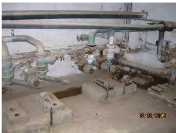
Figure 8. Air connection pipes
