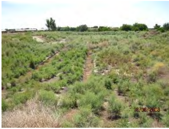
Figure 9. Sludge drying beds
