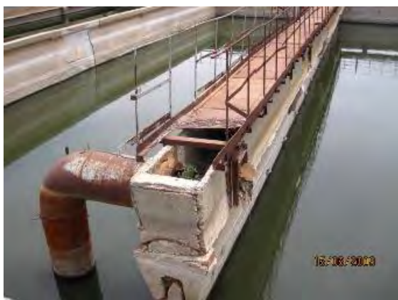
Figure 5. Aeration tanks (10,000 m 3 /day)
