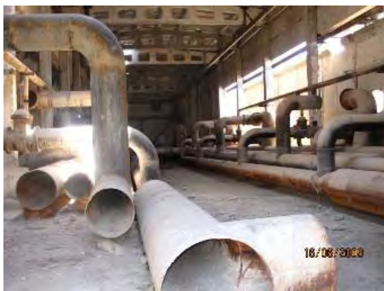
Figure 2. Uncompleted sand filter
