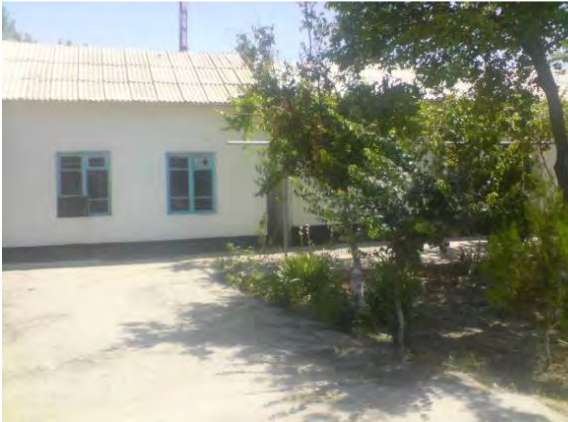
Photo 3. Office building of the Karmana District Vodokanal
