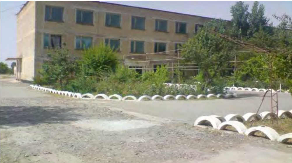
Photo 2. Office building of the "Kurpa" Water Distribution Unit of the Operational Directorate of Interregional Trunk Mains Damkhodja
