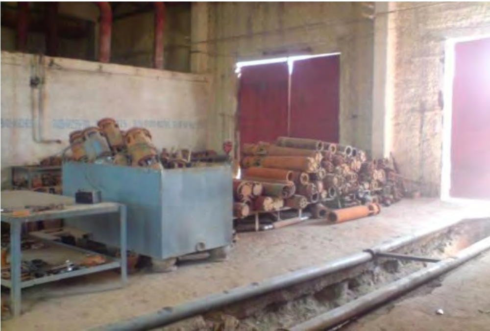
Photo 3. Workshop for repairing of pumps of the Water Distribution Unit “Kurpa”
