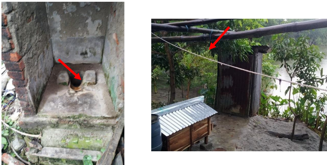
Figure 6: Containment technologies and their connections in Shariatpur. Left: Toilet Pit open to a nearby water body, Right: Toilet pipe connected to open environment (Source: Feasibility study 2020-21/DPHE)
