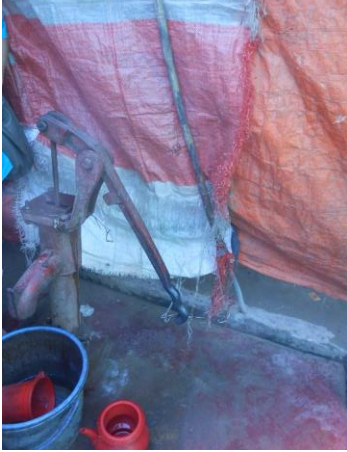
Screen placed by household in between water point and path in Camp 15
