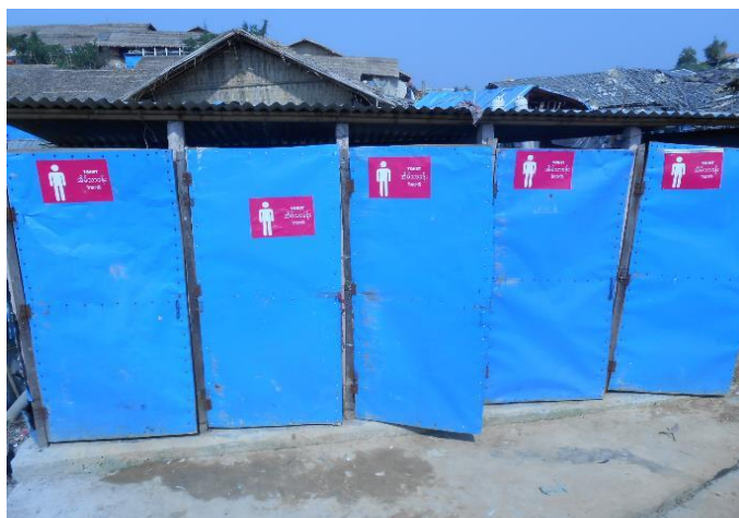
A block of male toilets constructed along a roadway (with no handwashing facilities)
