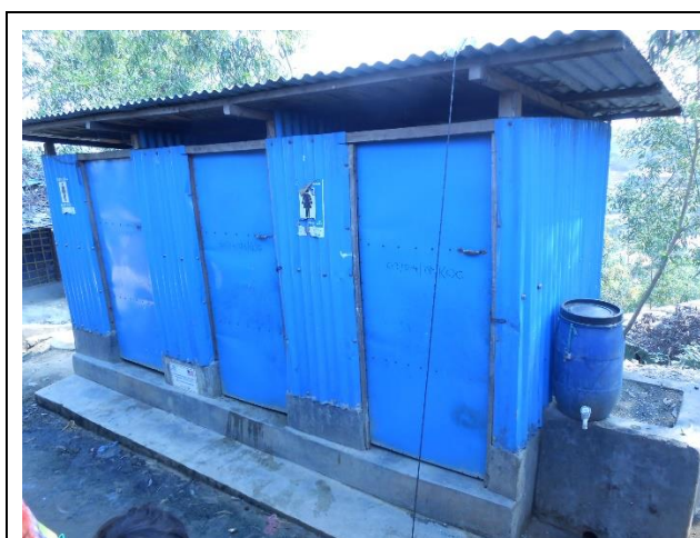
Latrine block in Camp 2 with handwashing drum present
