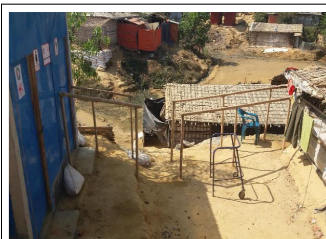
Handrails to entrance
