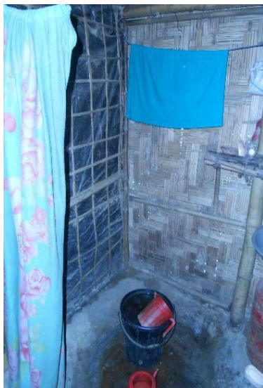
Self-constructed bathing facility inside a shelter next to the cooking area
