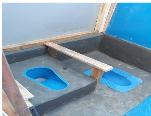
Two pans in one latrine – one raised for a person who cannot walk and moves across the floor
