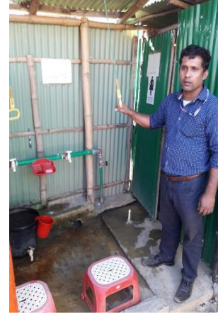
Accessible hand-washing facilities with stools and ropes with handles for an older person to help themselves sit and get up after sitting – in Age Friendly Space in Camp 18 supported by RIC/HelpAge
