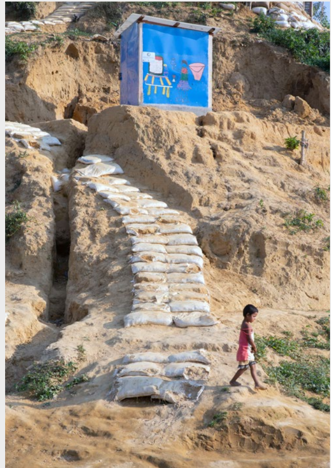
A latrine block up a hillside in Cox's Bazar, Bangladesh. Sandbags have been used to make steps up the hill, and to help prevent further erosion. Latrines such as these ones may be inaccessible to people who have difficulty climbing steps including older people, people with disabilities, pregnant women and young children. © Farzana Hossen / British Red Cross
