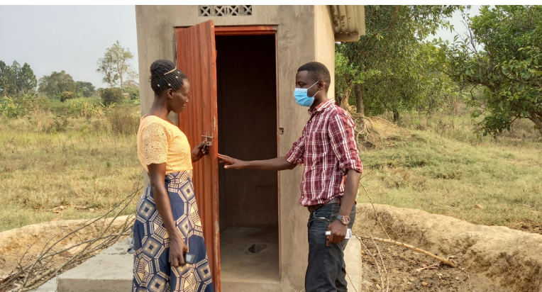
Inspection of a completed toilet.
