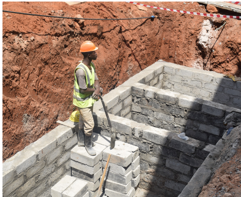
Masons constructing a septic tank.
