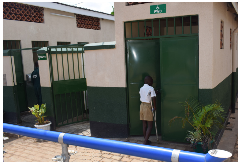
Pupil accessing an inclusive toilet for the disabled
