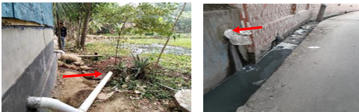
Figure 6: Containment technologies and their connections in Cumilla City Corporation. Left: Toilet pit open to a nearby water body, Right: Toilet pipe connected to open drain (Source: Feasibility study 2020-21/DPHE). containment and discharges directly to the environment (KII, FGDs, HH survey, 2020).
