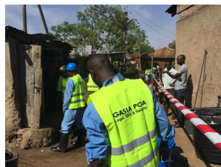
Figure 5 Workers equipped in PPE and easily identifiable
