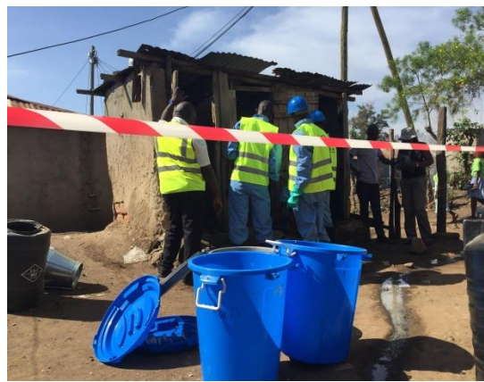
Figure 4 Barrier tape erected around work site
