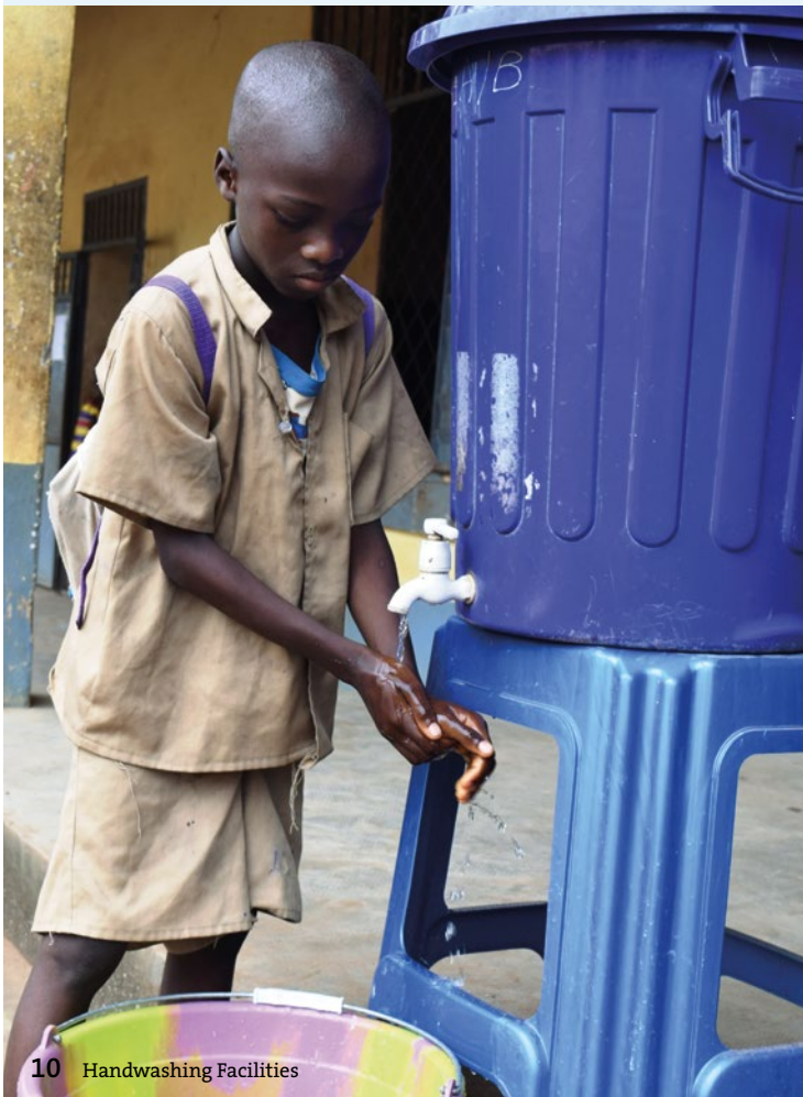
Facility on a school premise in Guinea: manually refillable, separate greywater bucket and tap with an extended handle. Source: GIZ Sector Programme Sustainable Sanitation, 2019.
