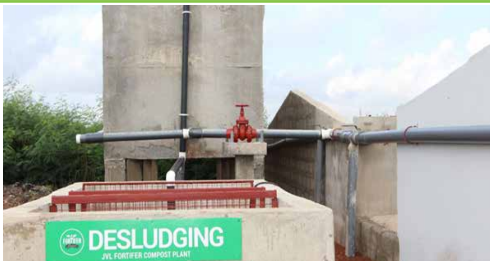
FIGURE 5. RECEIVING AND MIXING CHAMBERS OF THE 'FS FEEDING AREA' WITH A GRID FOR COARSE CONTAMINANTS.
