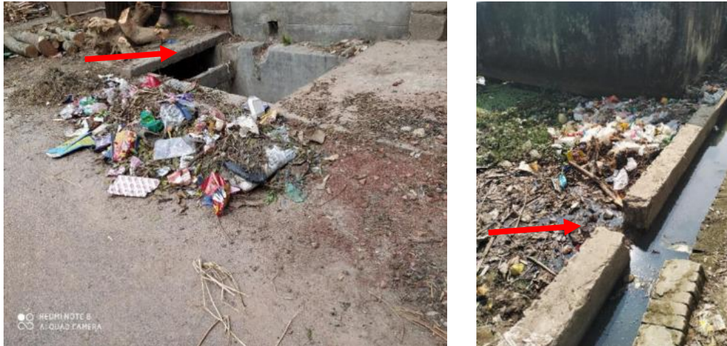
Figure 6: Containment technologies and their connections in Chuadanga. Left: Septic tank connected to the nearby water body. Right: Toilet pipe connected to open drain. (Source: Feasibility study 2020-21/DPHE).
