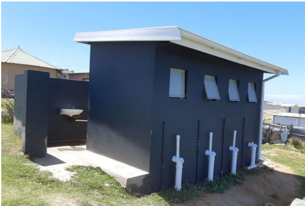
Figure 6: Well-maintained communal toilets
