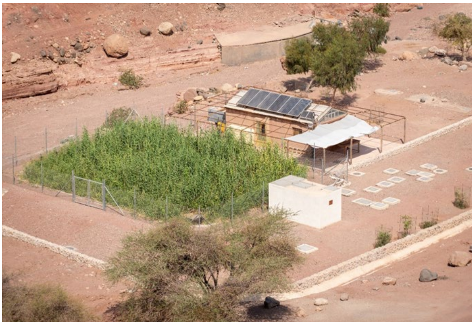
Figure 39 DWWTP at Feynan Ecolodge, Dana Biosphere Reserve
